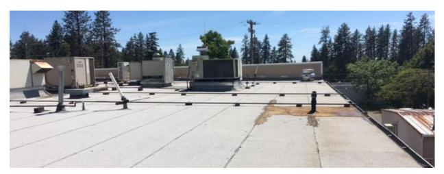
Following inspections by Public Works, Building, and local contractors, staff recommended the complete removal and replacement of the roof in-kind. The roofing material has adequate fall for drainage and is simply in need of regular replacement. As a result, staff has assembled the following project scope:
